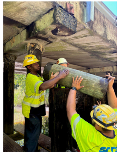
4) Splicing in new pile
