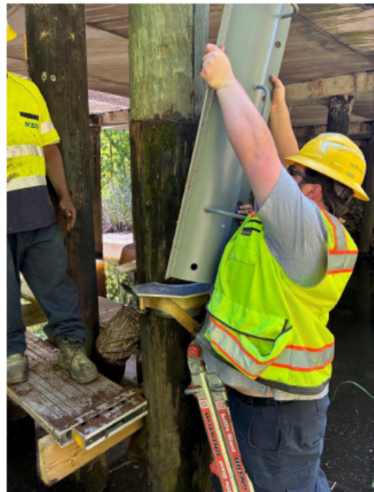
8) Placing Collar on Top Hat
