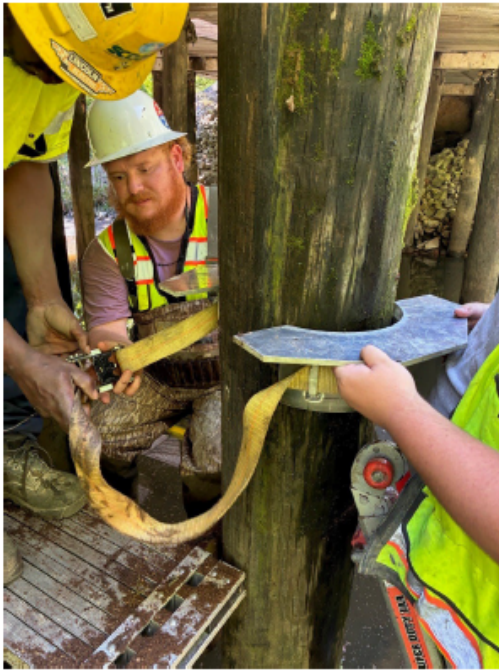
5) Installing Top Hat 2; below joint
