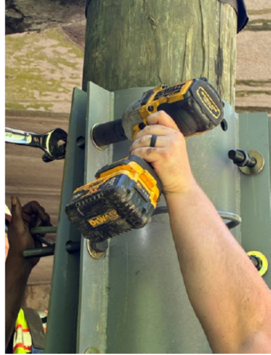
10) Tightening Bolts
