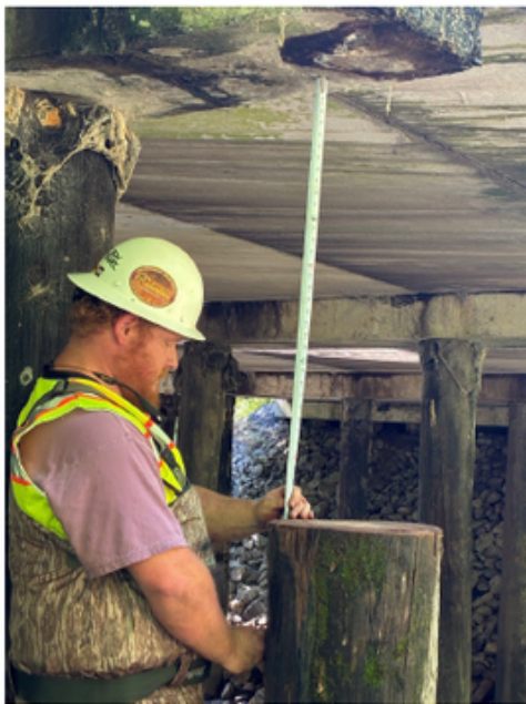
3) Measuring for new pile
