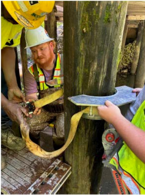
5) Installing Top Hat 2; below joint
