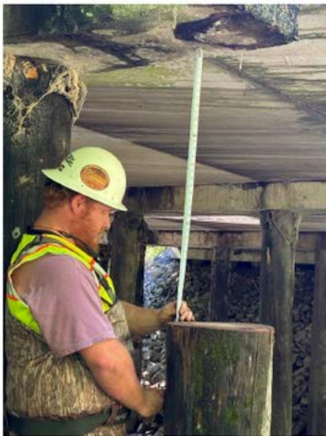
3) Measuring for new pile
