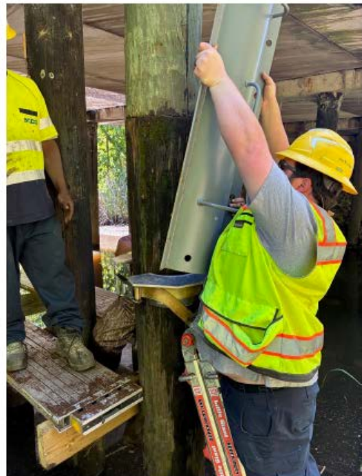
8) Placing Collar on Top Hat
