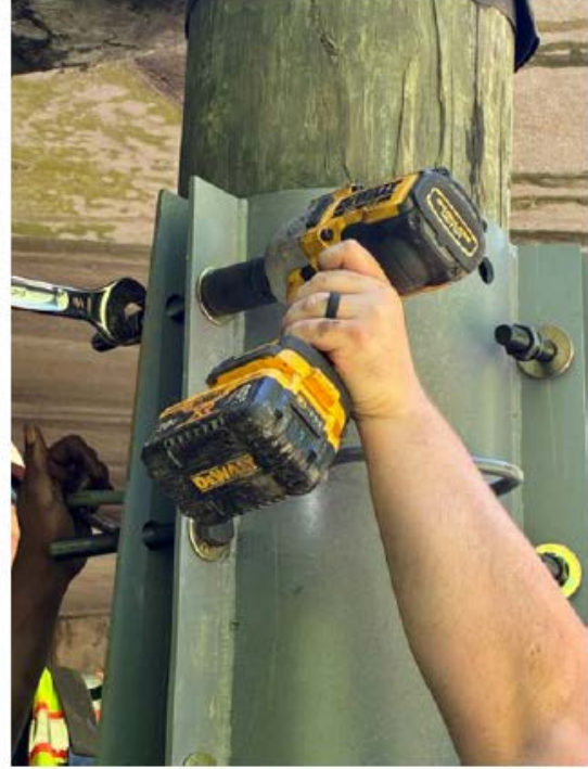
10) Tightening Bolts
