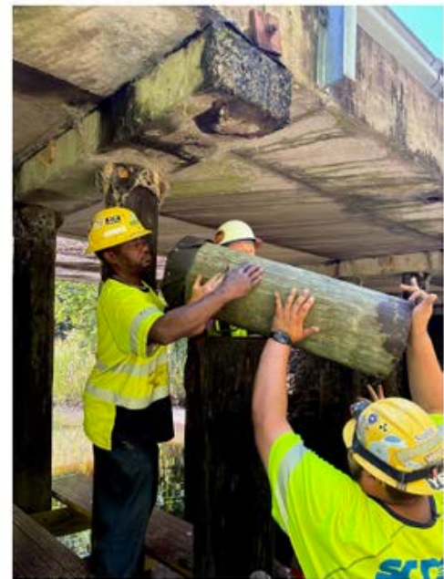
4) Splicing in new pile
